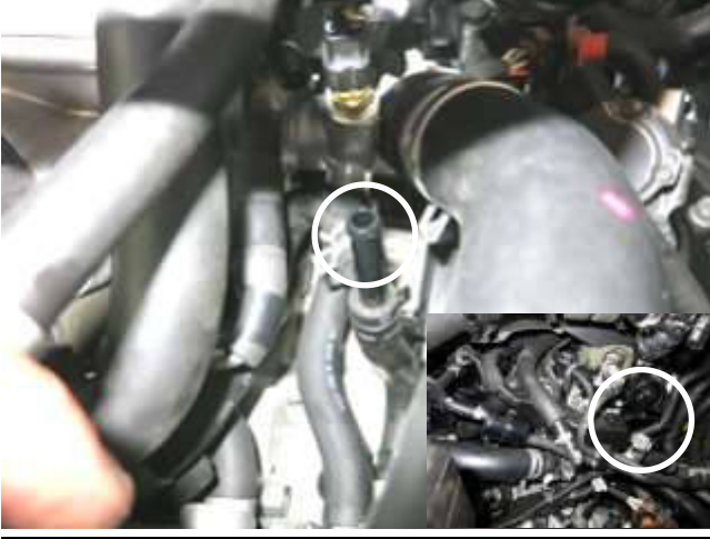
i. Route the previous hose above the “hard line” and too the “T” fitting. Connect the other end of the hose to the “T” fitting and secure with the spring clamp from step 2j. Then, with the two provided vacuum caps, cap the ends of the hard line.
