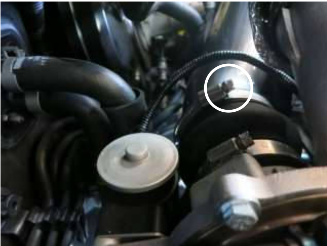
m. After proper tube alignment is achieved, tighten the hose clamp around the tube at the turbo.
