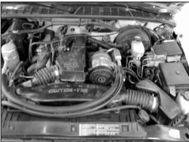
Factory air box system installed
