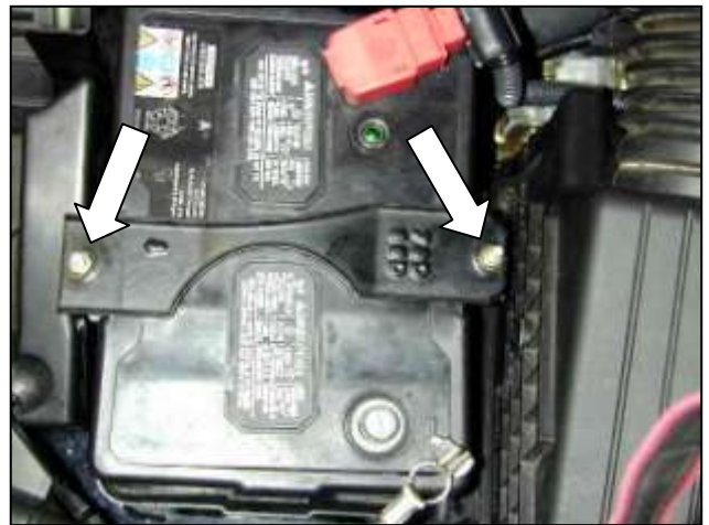
b. Remove the battery tie down bracket and the J bolts that hold it in place. Disconnect the positive battery terminal.
